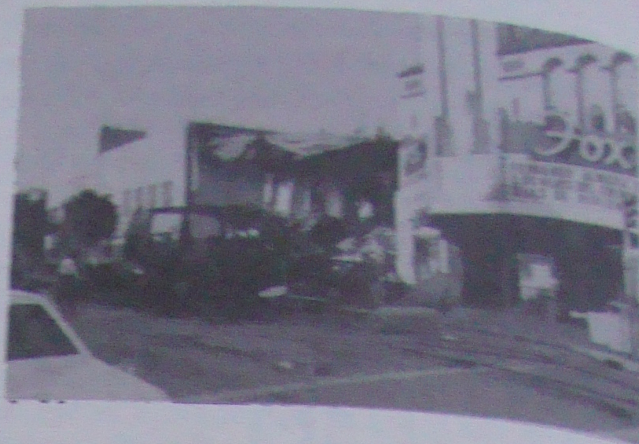
Fig.4 Collapsed unreinforced masonry building in Watsonville
