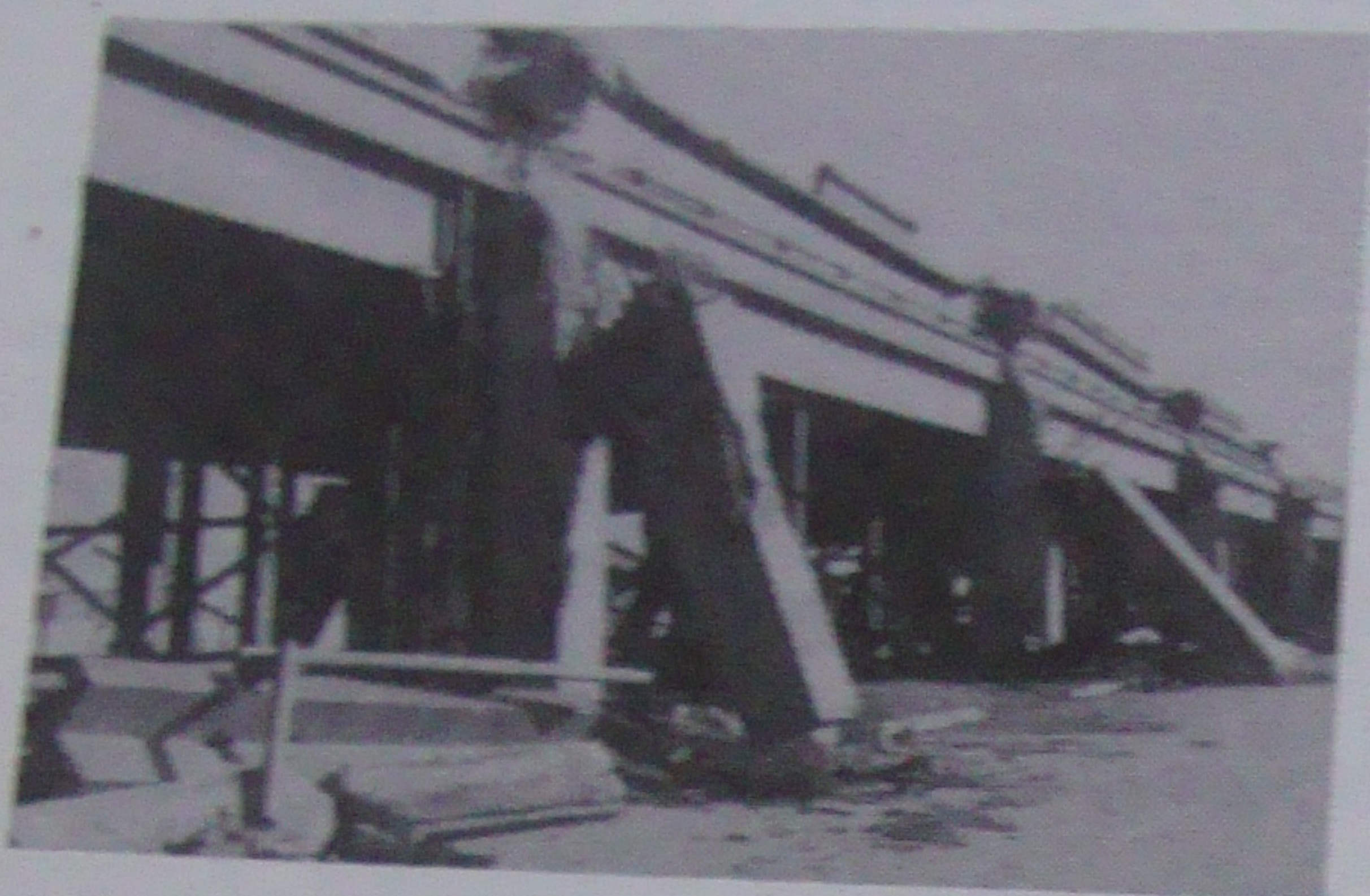
Fig.5 Collapsed Nimitz viaduct of I-880
